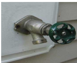
Hose bib without BFP; water supply is susceptible to contamination when a hose is connected.
